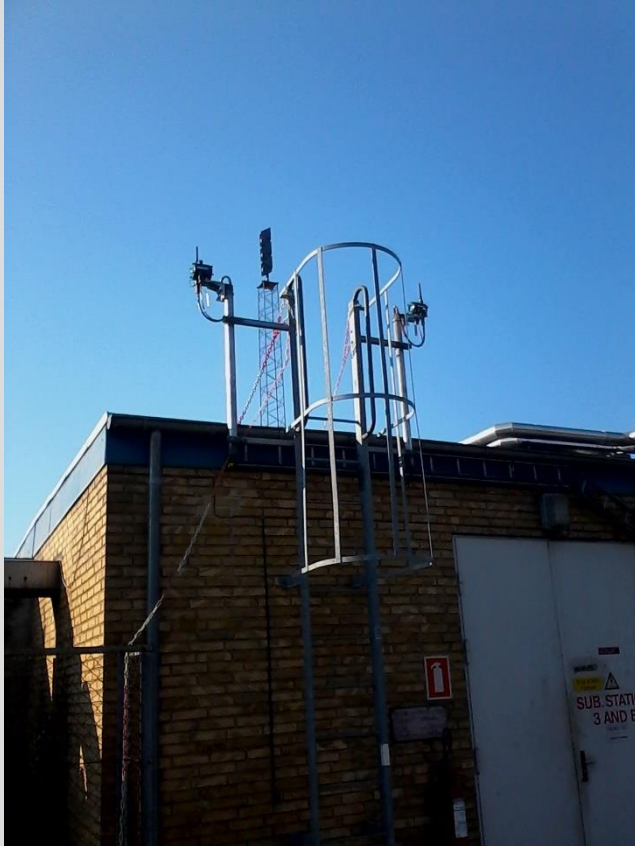
Dual access points with good access to a majority of the detectors.
